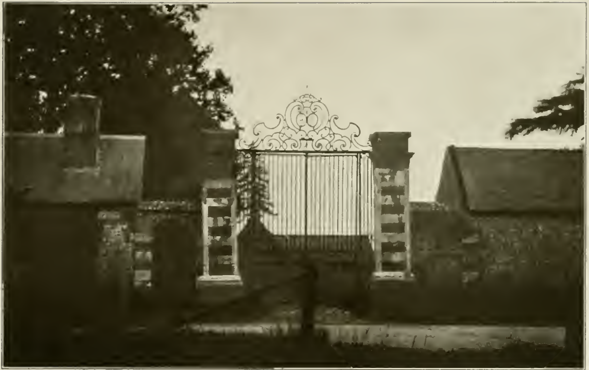
PLATE 160. Farm gate near St. Jean-de-Follerville, Seine-Inférieure
